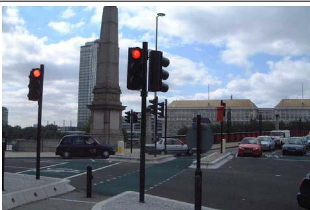
**Photo 6.2** Exclusive signal controlled cycle crossing. *Courtesy CTC*
