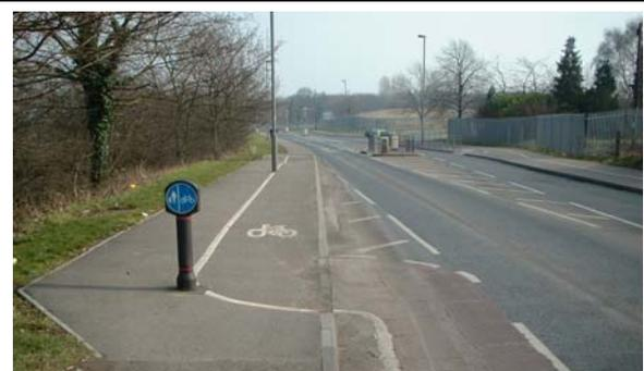
**Photo 5.11** Cycle lane leaving the carriageway to join a cycle track on a segregated footway.
