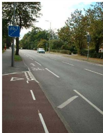
**Photo 5.8** Shared use cycle track joining a cycle lane. Note use of hatching to push vehicles out and protect cyclists.
